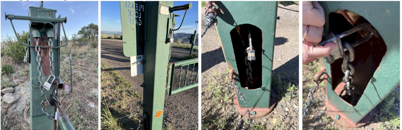
Chain closure on west face of post with authorized locks
