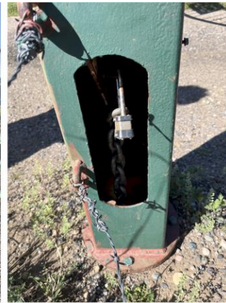
East face of post
